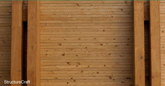
Nail-Laminated Timber
