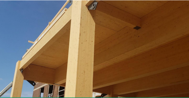
Glue-laminated Timber (Glulam)
